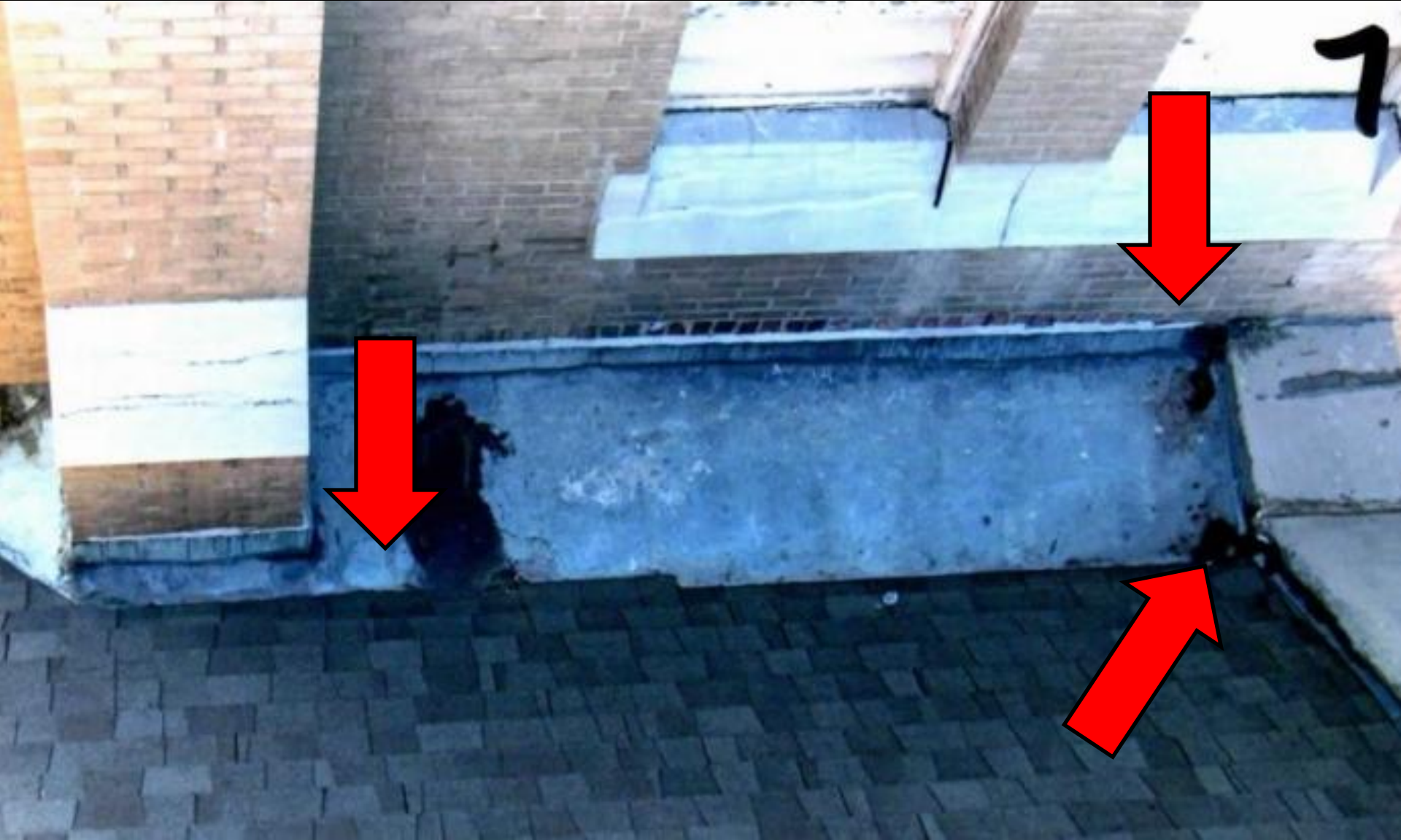
Roof valleys, flashing
